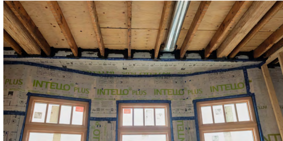
Top Left: Sealing around floor joists
