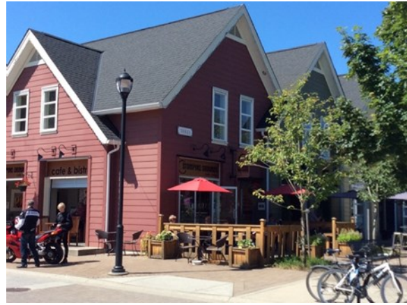
Figure 42. Commercial open to the street, incorporating patio space, landscaping and nearby bike parking.
