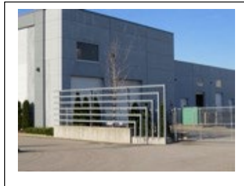
Screening of service and loading areas
