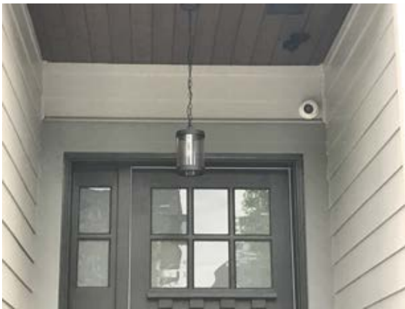
Use energy efficient lighting with motion sensors to avoid unnecessary use.
