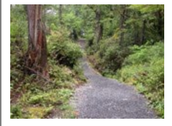
Trail with 2.5 metre width and 250 mm shoulder
