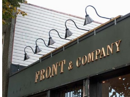
Figure 47: Gooseneck lighting highlights signage and directs light.
