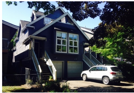
Figure 18: Example of a duplex that reduces the prominence of front vehicle access and garage by emphasizing the entrance and verandah.
