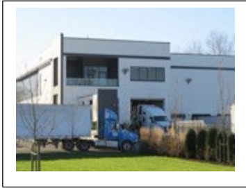
Loading and service bays to the side and rear of the building
