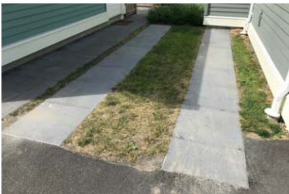
Utilize permeable paving materials or use of parking strips to reduce paved areas and increase absorption of water run-off.
