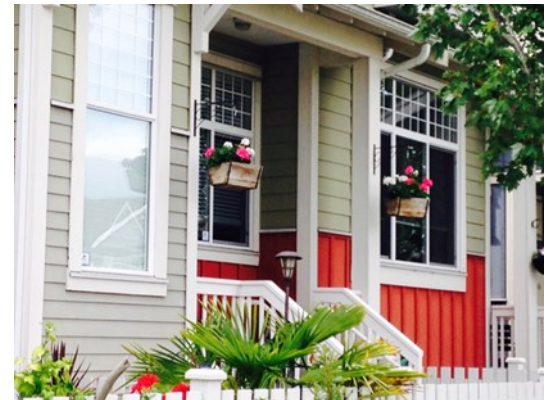
Figure 29. Multi-family development with a small verandah, overhang, and use of horizontal wood siding.
