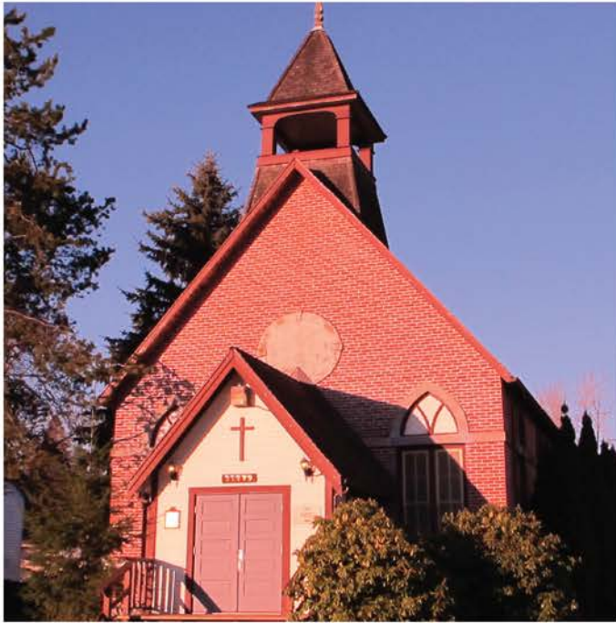
SAINT ANDREW'S PRESBYTERIAN CHURCH 22279 116 Avenue 1888
