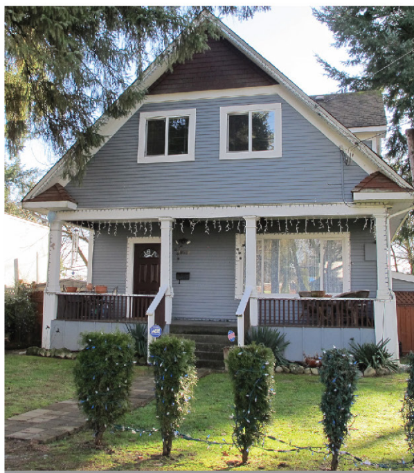
PATTERSON RESIDENCE 20582 113 Avenue 1912-13
