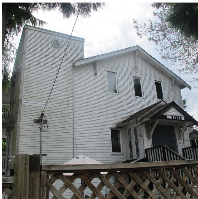
MAPLE RIDGE BAPTIST CHURCH 21390 Dewdney Trunk Road 1912
