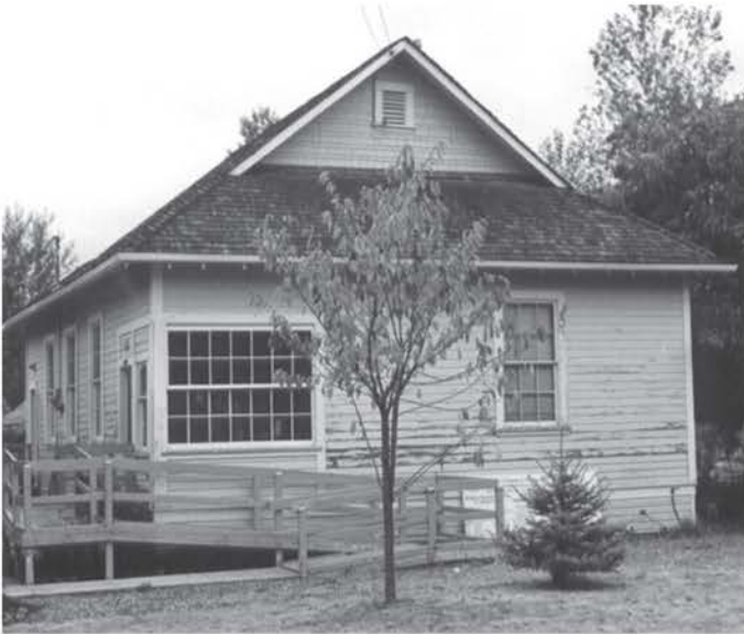
Kindergarten Building, 1998 Inventory
