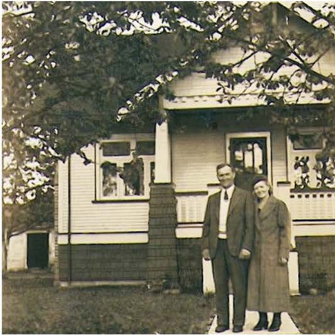
Neighbours visiting the Whitehead Residence.
