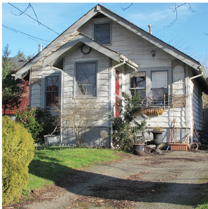
WILSON RESIDENCE 11252 Dartford Street 1937
