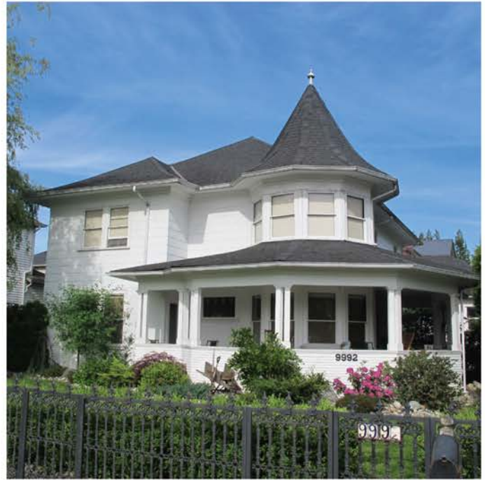
HILL HOUSE 9992 240 Street 1912
