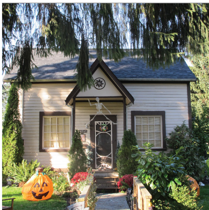
JOHN HAMMOND HOUSE 20541 Lorne Avenue 1891-92
