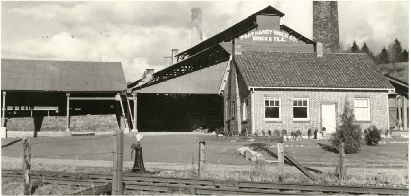
Port Haney Brick Co. Office [MRMA P00958]
