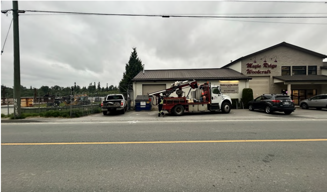
Photo 1 Drilling at location BH25-01/SCPT25-01. Facing south.
