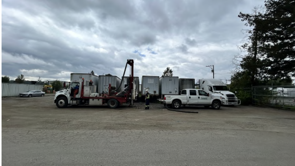
Photo 3 Drilling at location BH25-03/SCPT25-03. Facing southwest.
