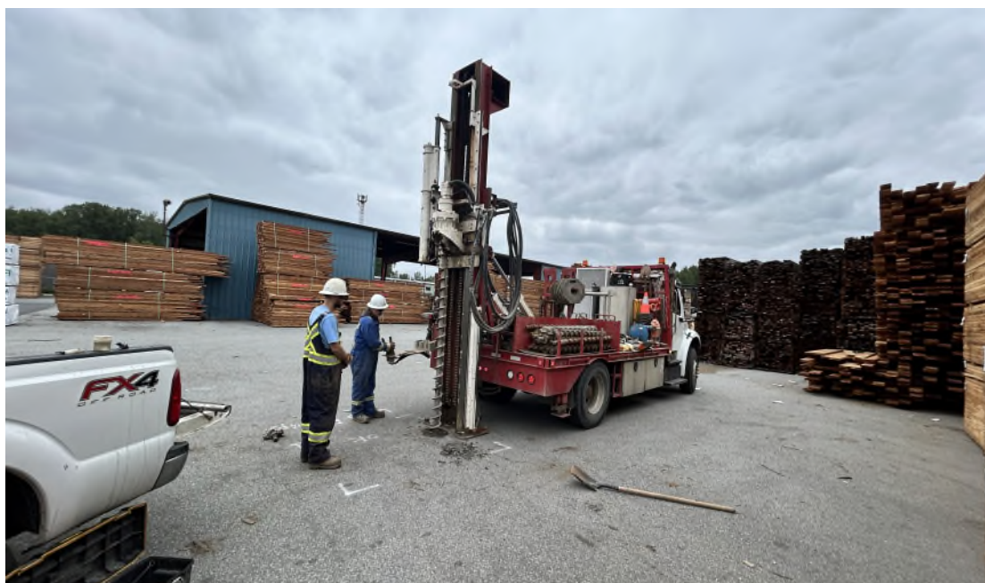
Photo 6 Drilling at location BH25-05/CPT25-05. Facing northeast.
