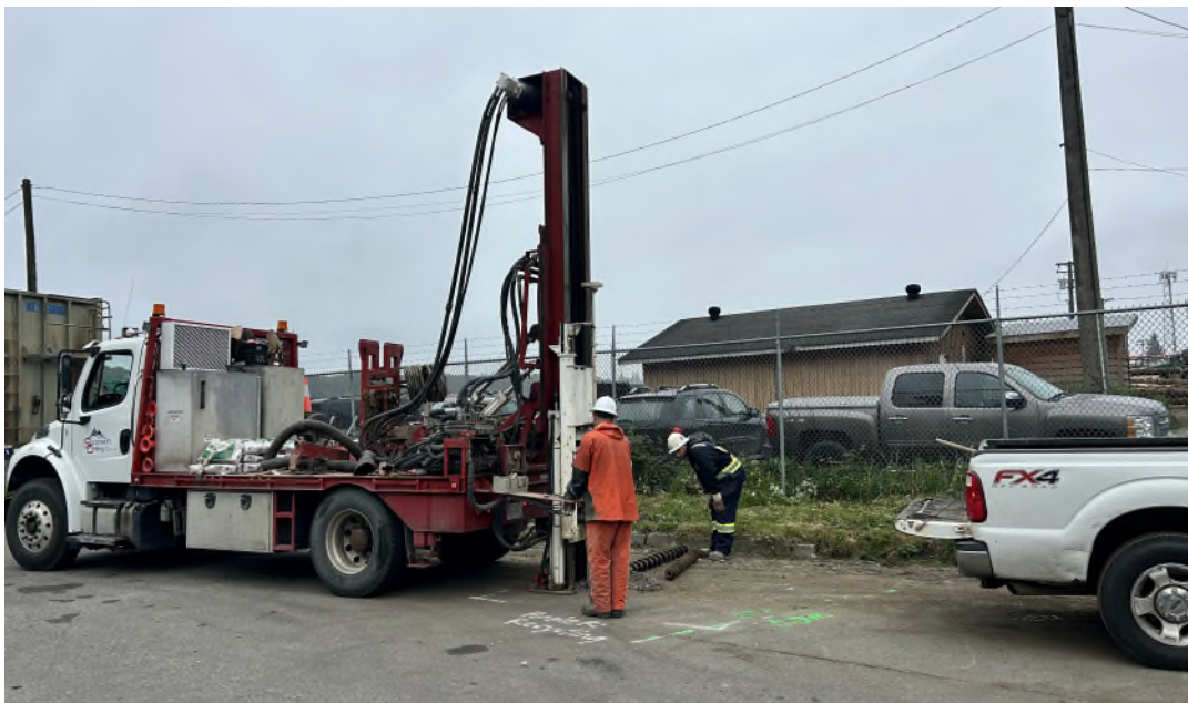
Photo 2 Drilling at location BH25-02/CPT25-02. Facing northwest.
