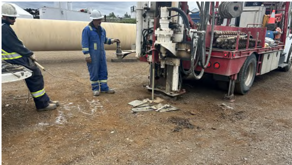
Photo 4 Drilling at location BH25-04/CPT25-04. Facing south.
