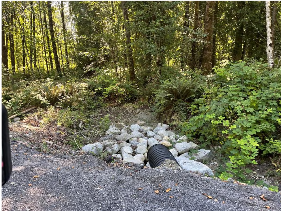
Photo 42: Culvert draining settlement pond on south portion of 25927 128 Avenue
