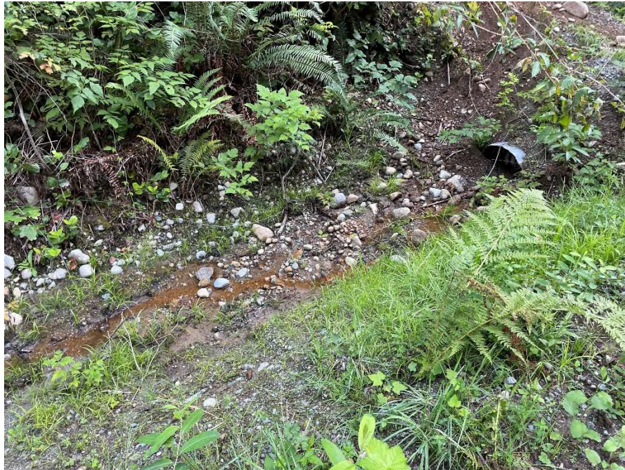
Photo 6: Unmapped drainage ditch culvert parallel to Frodo Creek, north view.
