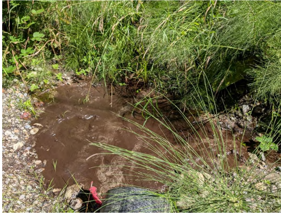
Photo 21: Culvert at mapped stream east of 249 Street.
