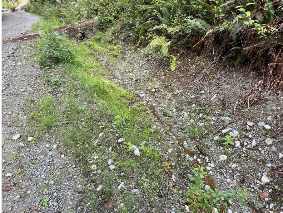
Photo 7: Unmapped drainage ditch culvert parallel to Frodo Creek, south view.
