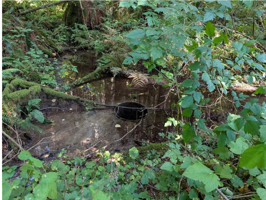
Photo 27: Mapped culvert, non-fish passable, east of 249 Street.
