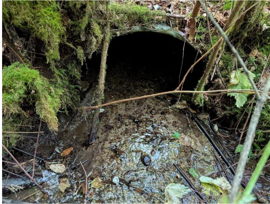
Photo 19: Unmapped culvert and unmapped 249 Street Creek.
