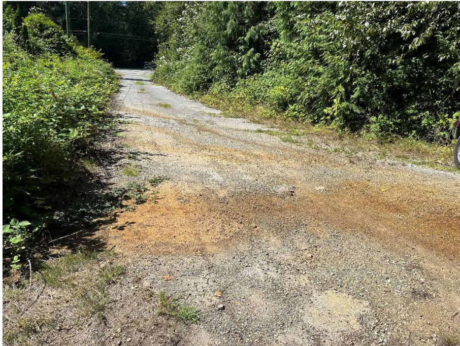
Photo 36: Iron staining, possibly from past flood events, on north side of 13120 256 Street
