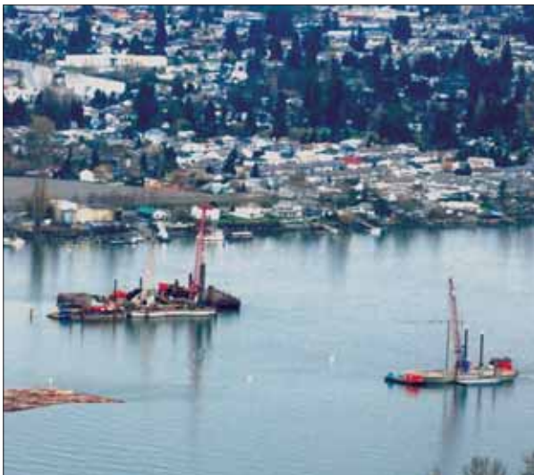
Golden Ears Bridge construction
