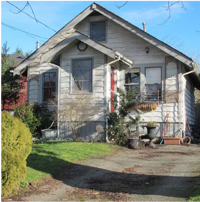
WILSON RESIDENCE 11252 Dartford Street 1937
