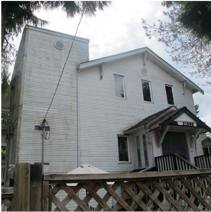
MAPLE RIDGE BAPTIST CHURCH 21390 Dewdney Trunk Road 1912
