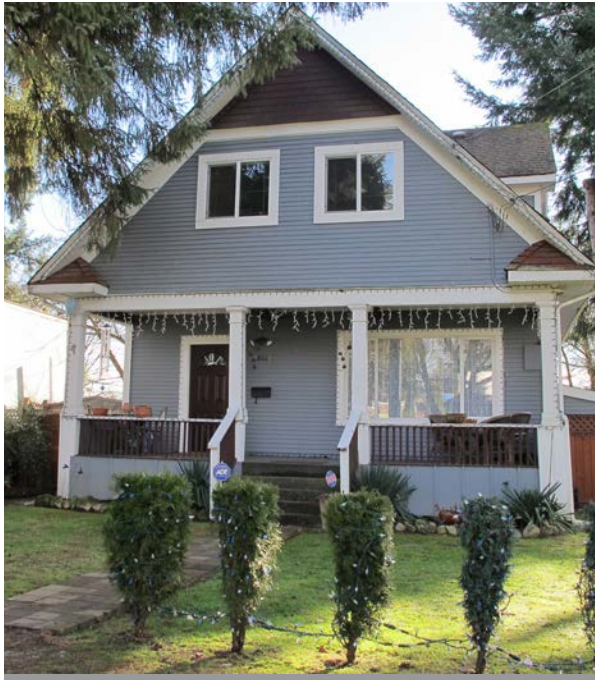
PATTERSON RESIDENCE 20582 113 Avenue 1912-13
