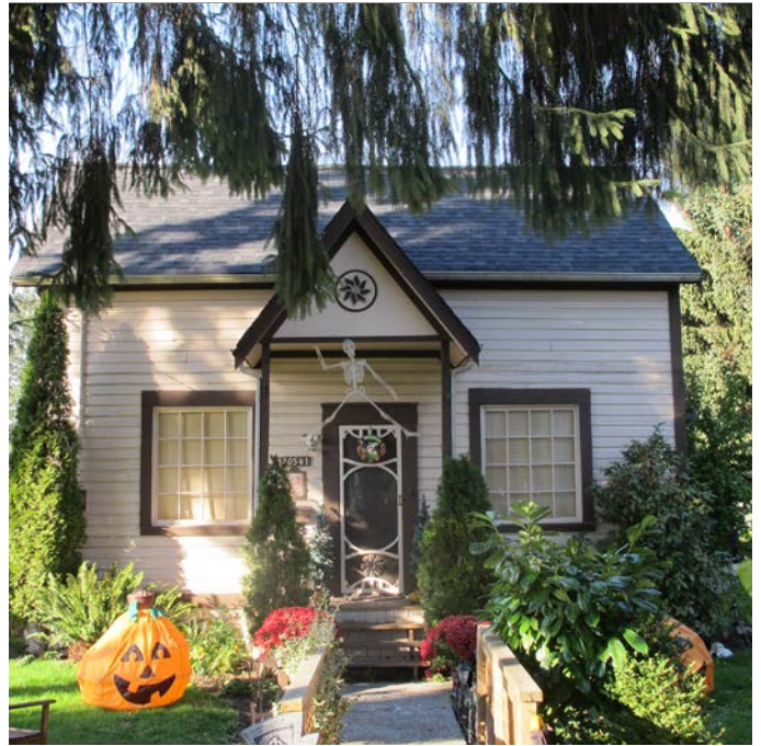
JOHN HAMMOND HOUSE 20541 Lorne Avenue 1891-92
