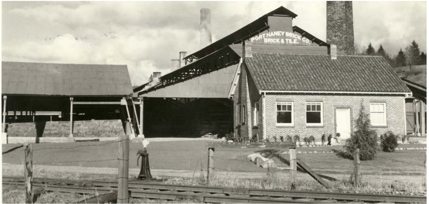
Port Haney Brick Co. Office [MRMA P00958]
