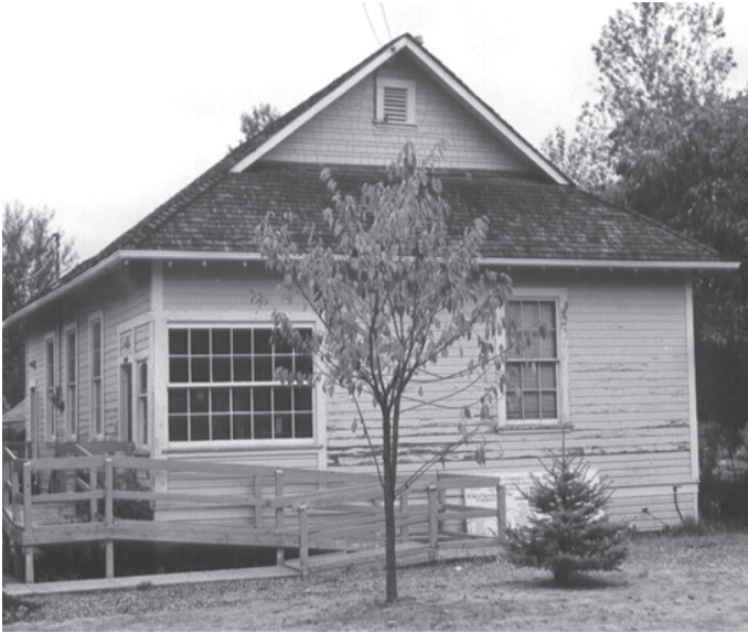
Kindergarten Building, 1998 Inventory
