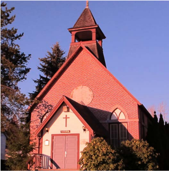
SAINT ANDREW'S PRESBYTERIAN CHURCH 22279 116 Avenue 1888
