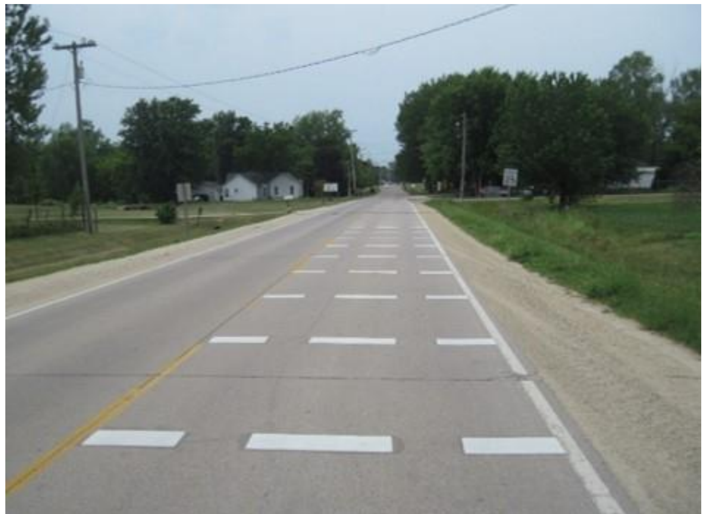
*Actual implementation may look like this with 2 small gaps for wheel path consideration
