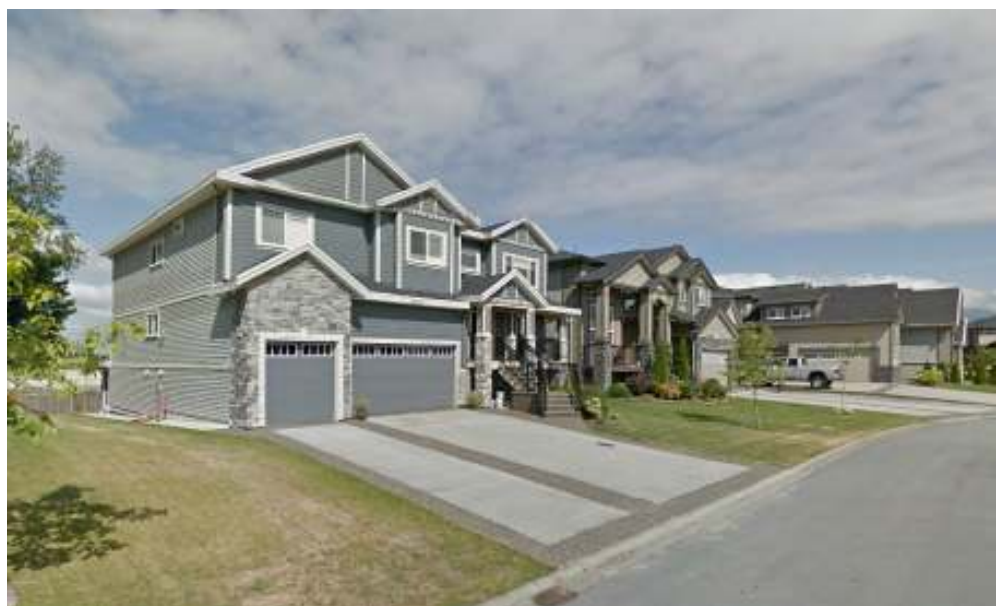
Photo at Right: Floodplain Construction in Maple Ridge
