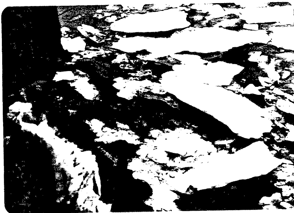
Photo 12. Evidence of launched riprap from same location as previous 3 photos.
