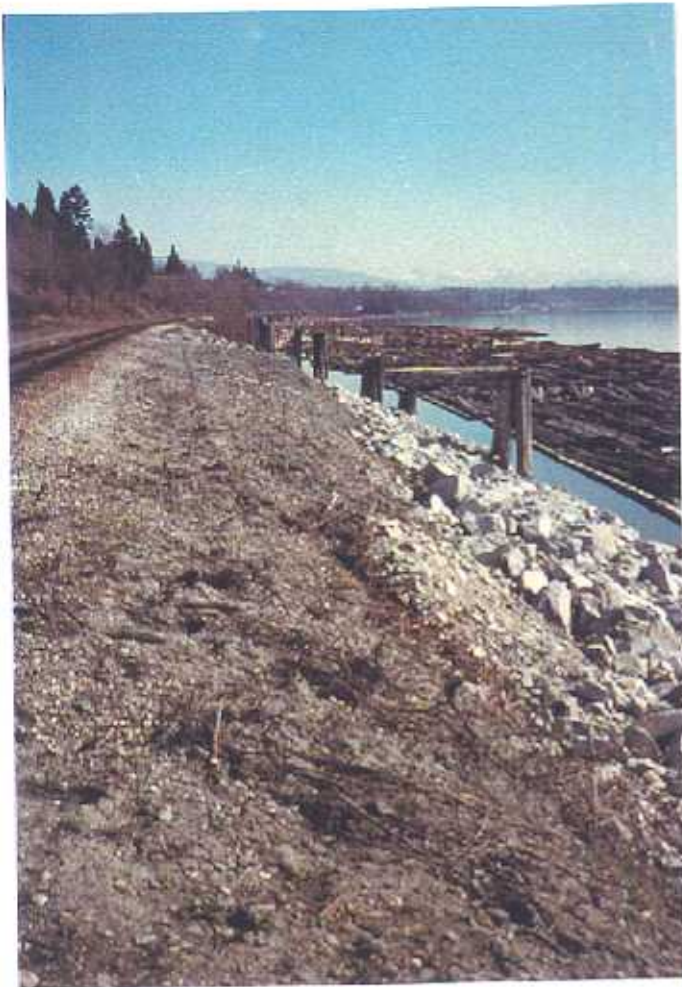
Photo 3: Rip-rap protection on riverbank slope below CPR tracks.
