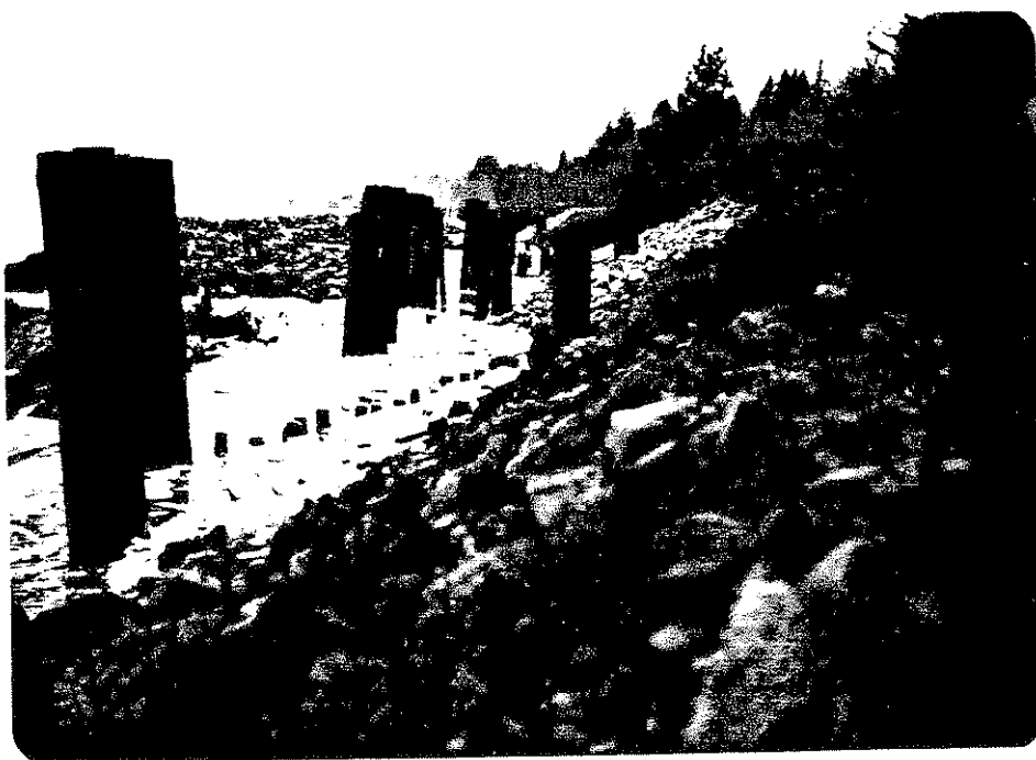
Photo 13. Another view upstream, a short distance upstream of photo 12. Riprap in this area has been placed for some time. Note old piles cut off above low water line at left. Also, looking upstream note intermittent placement of riprap.
