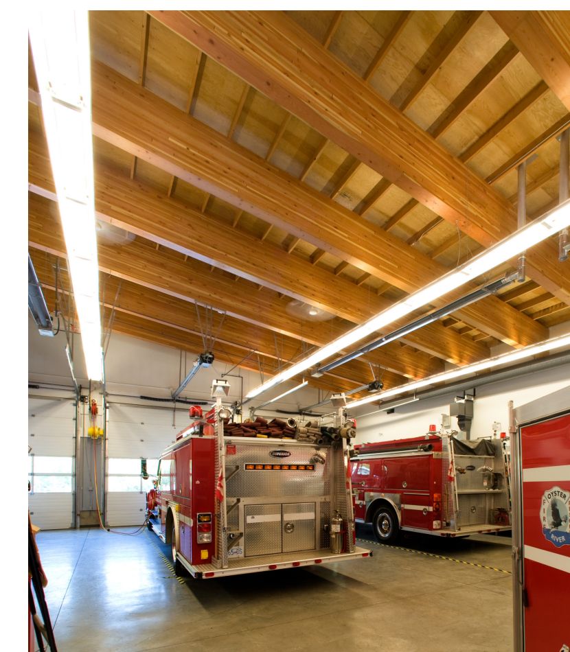
glulam beams in apparatus bays
