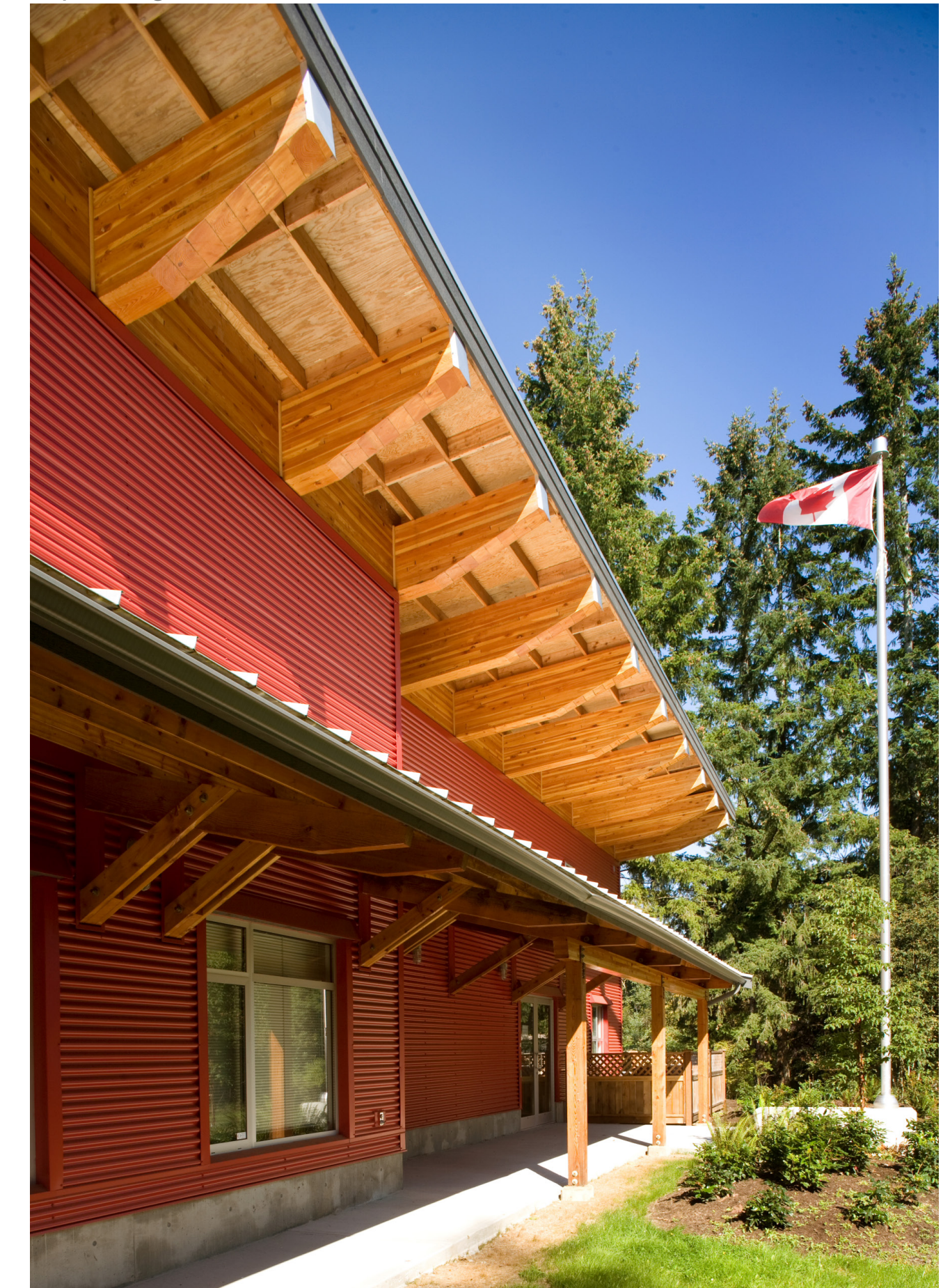
exposed glulam beams at exterior
