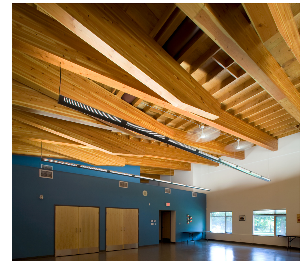
exposed glulam beams and wood ceiling in training room
