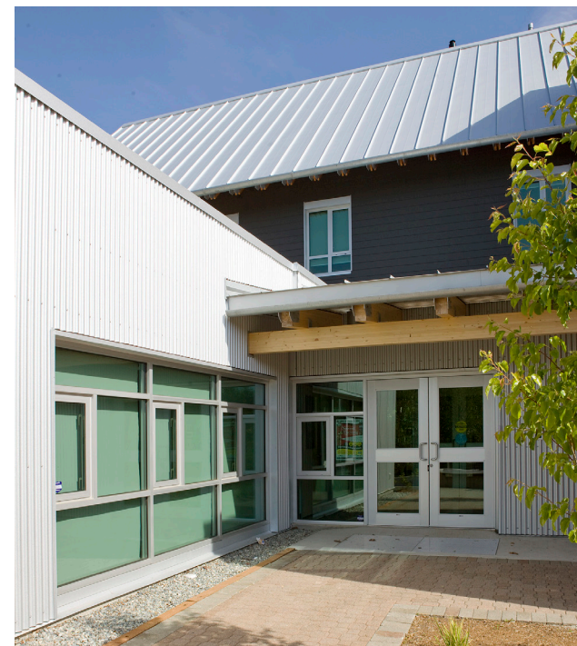
standing seam metal roof (weather zinc colour)
