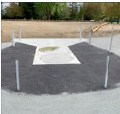
Construction is progressing to replace the previous throws area with a competition level Hammer and Discus Throws facility. The work completed includes leveling the grass field, installing a small retaining wall, and new drainage system.
