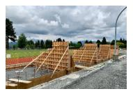
Work continues on several projects at Maple Ridge Secondary School. The new bleacher building is starting to take shape, formwork is in progress with plans to pour concrete later this week. Underground rough-ins for plumbing are complete, and
