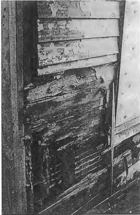
Gillespie Residence Front Entrance Rot Condition At North Side of Front Door
