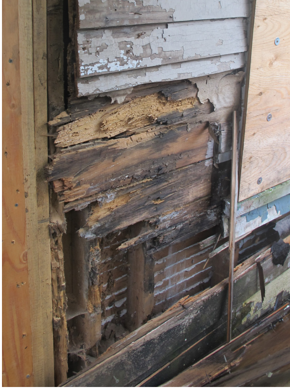
Gillespie Residence Front Entrance Rot Condition At North Side of Front Door
