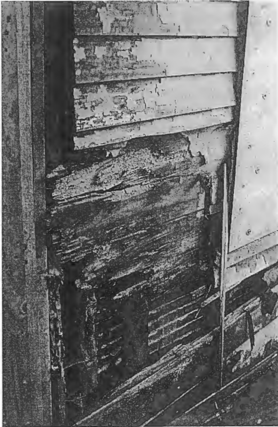
Gillespie Residence Front Entrance Rot Condition At North Side of Front Door
