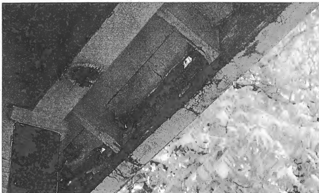
Gillespie Residence Front Entrance Rot Condition At Soffit and Trim Board Interface.
